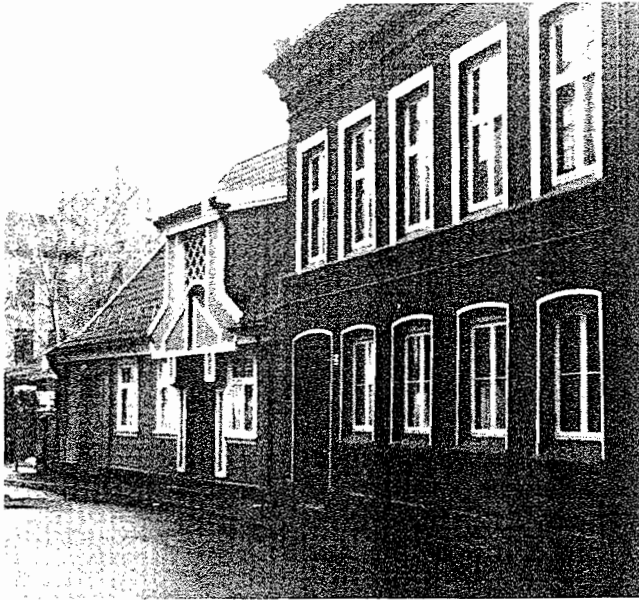
Diocesan offices etc at Akersveien 12 and 14, ancient houses newly renovated.
